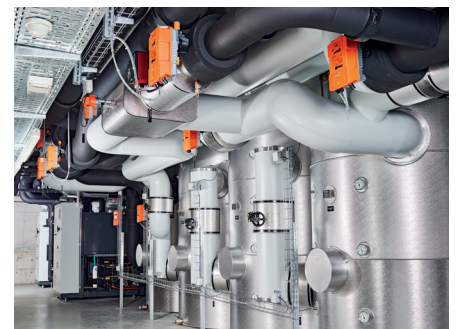
Butterfly valves with PR actuators ensure the correct flow rate of the heating and chilled water in the main distribution.
