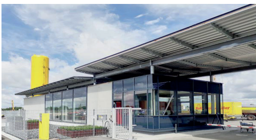
Picture of the power station at Müller Produktions GmbH in Ungerhausen near Memmingen (DE)
