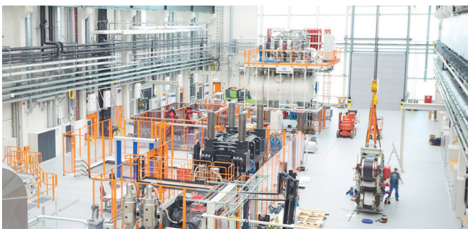
In the middle of the OHLF building, with an area of 2'100 m 2 , is the technical centre.
