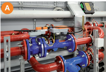
The Challenger site with the application areas of the Belimo Energy Valve™ in the cooling and heating circuit
