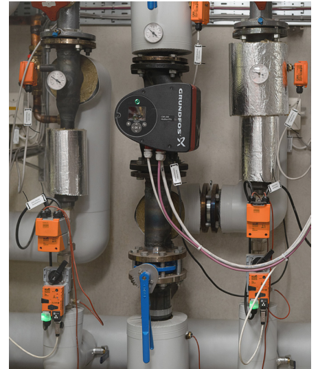
Injection Circuit with 2-way Belimo Energy Valve™
