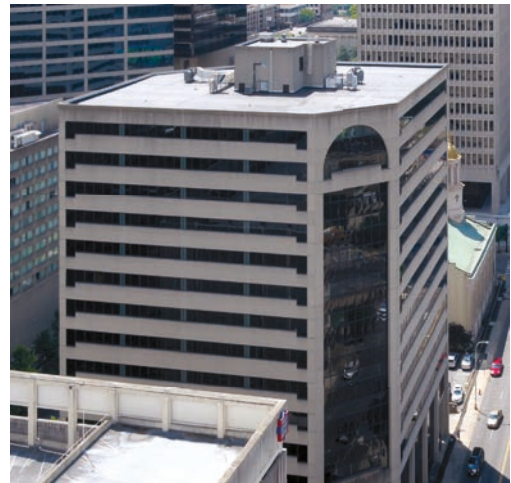
Abb. 72: Tennessee State Office Building.
