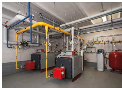
Abb. 113: Condensing gas boiler
