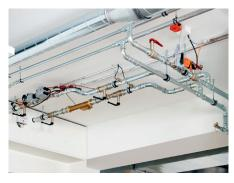
The electronic differential pressure valve EDPV is a control valve that ensures constant inlet pressure in the zones' ring pipes and communicates with the Belimo Cloud as IoT components.
