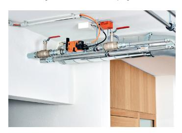
The 2-way characterised control valve with IoT rotary actuator which the condensation sensor is directly connected to, enables very easy integration into the controller.
