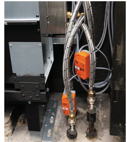
Top left: Old unit. The new units (bottom left as the master) are now regulated on the primary air side and water side (right) by the Belimo actuators.
