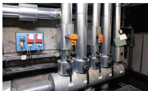
The proven standard Belimo globe valve actuators are also used with the flange valves of the new air handling units in the GENO-Haus building.
